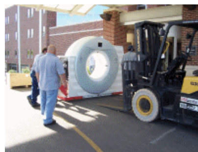
Specialists with Siemens Medical Solutions install the new 64-slice computerized tomography (CT) scanner at Bothwell Regional Health Center.
